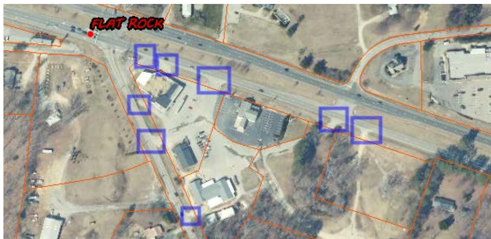
Figure 1: Access Points Prior to Redevelopment
